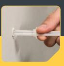
Zip the nylon collar towards the wall so the collar sits into the drilled hole. Then snap off the nylon arms.
